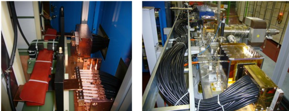
<Figure 2.1.4.48> 20 coaxial cable strands in parallel connection.
