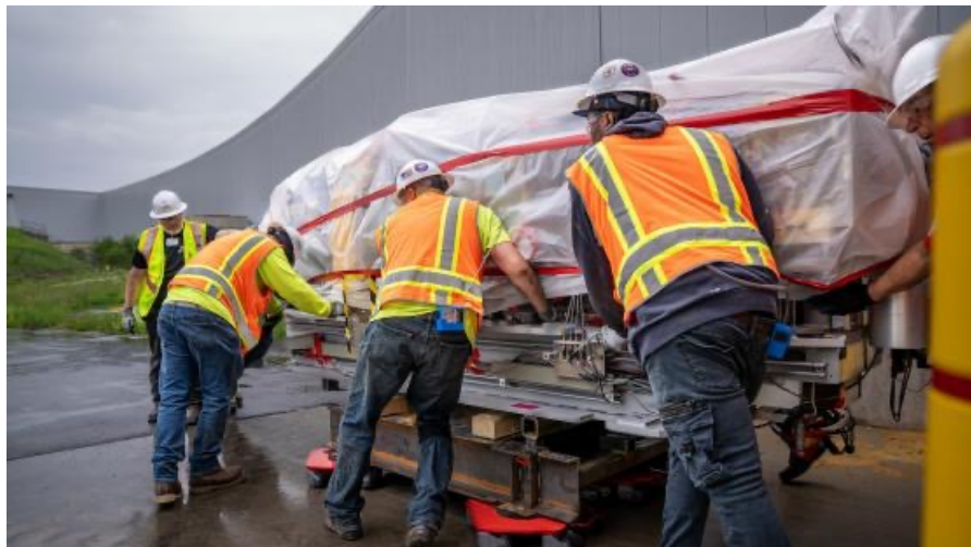
First girder of old APS storage ring coming out of ring in May, 2023
