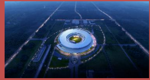
Hefei Advanced Light Facility
