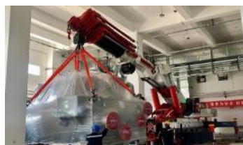
Apr. 13, 2021 Utility installation in NO.2 Hall commenced
