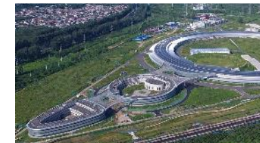
Nov. 3, 2023 Civil Construction for ancillary buildings completed
